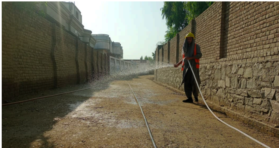
Dust control at the subproject sites in Jalalabad City - 24 Aug 2025
