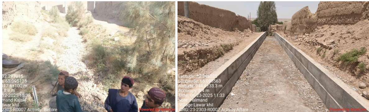
Before and After pictures of Drainage Canal in Lawar Khil in in Helmand Province, June 2025 @FP/CHA
