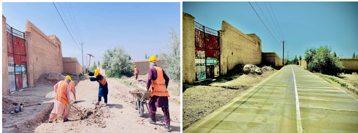
Before and after photos of a plum concrete surface tertiary road handed over to the community for use in Gozar #15, District #2, Gardiz City on 21 August 2025 (hand over date) @UNOPS
