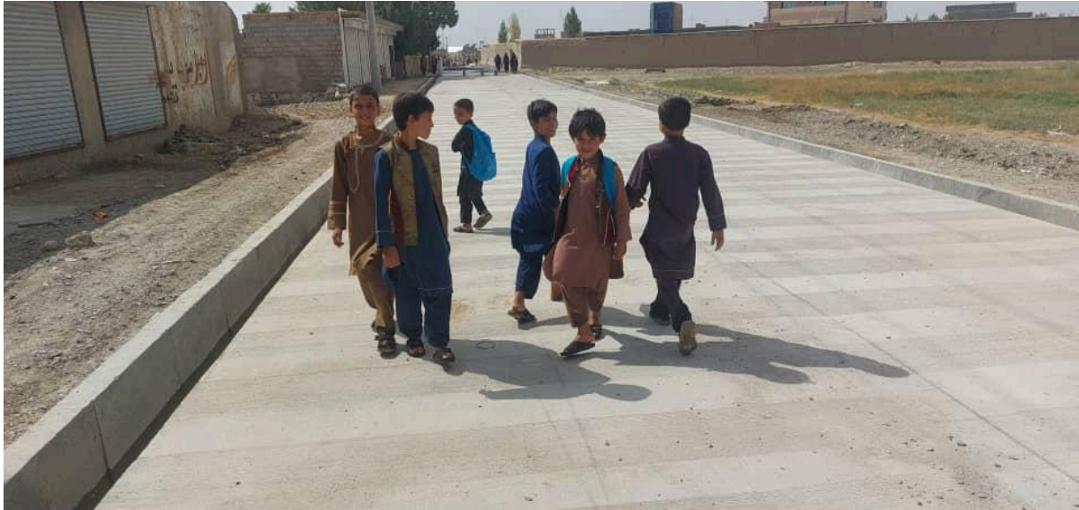
School children are benefiting from improved access through the Wahdat Abad plum concrete surface paved street with total length 520 m, Gozar 6 # District# 5, Ghazni City, 15 August 2025 @UNOPS
