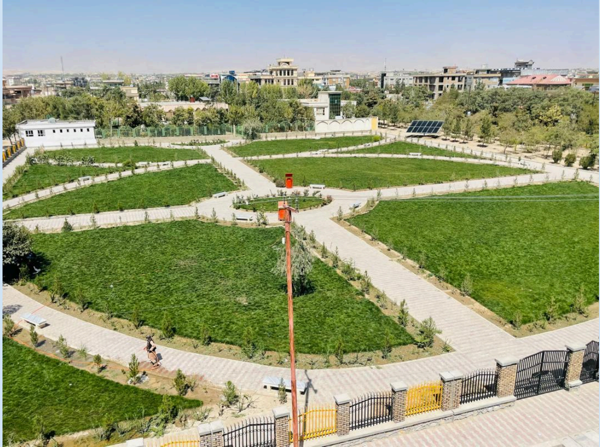
The same disused plot in Gozar 2, District 3 of Ghazni City after CRLP intervention, August 2025 @UNOPS/Rafiullah Hemat
